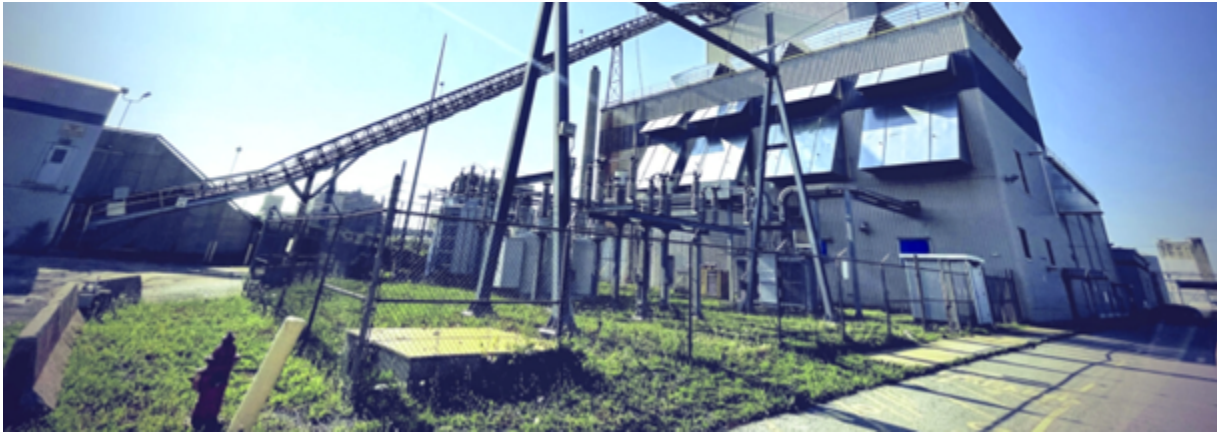
Figure 2 - Blockfusion's State-of-the-Art Datacenter, Converted from a Decommissioned Dirty-Coal Power Plant.
