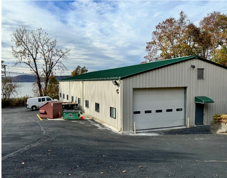
Figure 1 – Image of Exterior of NANO Nuclear's New Advanced Demonstration Facility for Key Components of its Nuclear Microreactor Designs in Westchester County, NY
