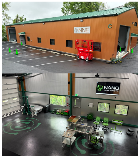
Figure 1 - Image of Redeveloped NANO Nuclear's Demonstration Facility for Key Components of its Nuclear Microreactor Designs in Westchester County, NY.
