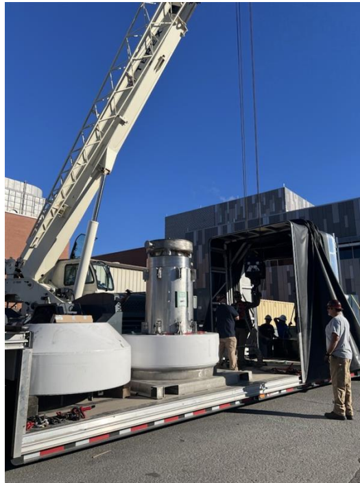
Figure 2 - Unloading a large cylindrical shielded cask for radioactive material transport or handling.
